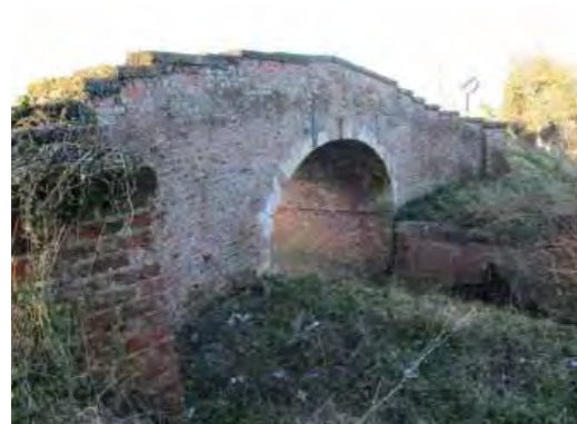
Photo 9: Strensall New Bridge
