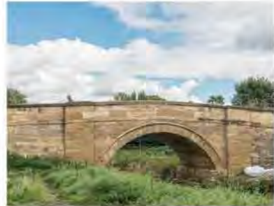
Strensall Bridge - Sheriff Hutton Road
