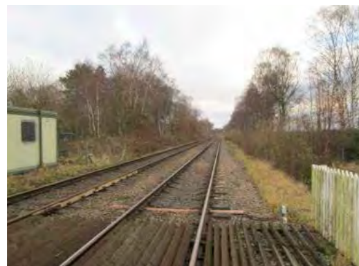
Photo 3: View of the railway line
