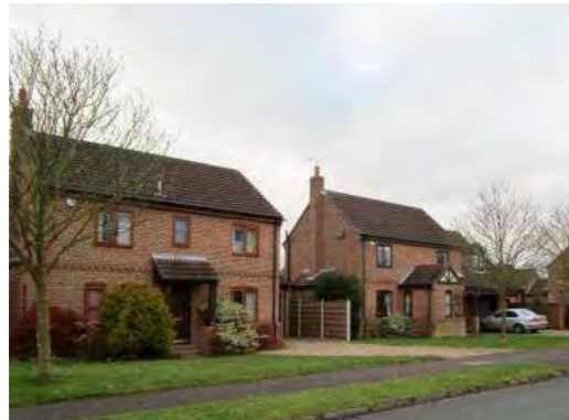
Photo 25: Twentieth century two storey housing
