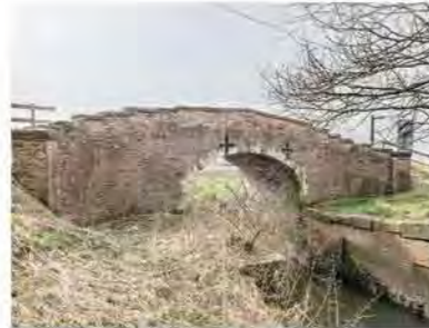
Strensall New Bridge - Haxby Moor Road
